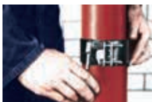
5. Alternatively tighten the two clamping screws uniformly and hand tight. The guiding and threaded plates of the clamp must come together parallel to avoid any deformations
