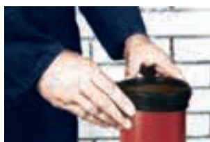
2. Turn over the open half of the sealing collar
