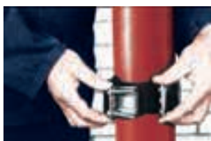
4. Place the clamping sleeve around the collar
