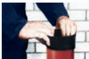
1. Push the supplied complete connector on to the pipe end right up to the middle spacing ring of the seal
