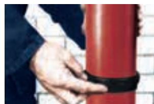
3. Install the next pipe or formed part flush with the spacing ring and fold back the turned over half of the collar
