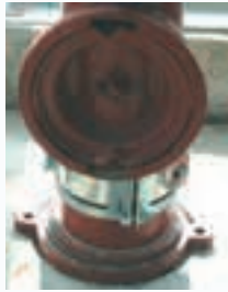
Resting on slab
